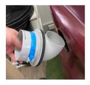
An overflow incorporating 316 stainless mesh with less than 1mm openings is required to ensure there are no entry points for mosquitoes or other vermin.
